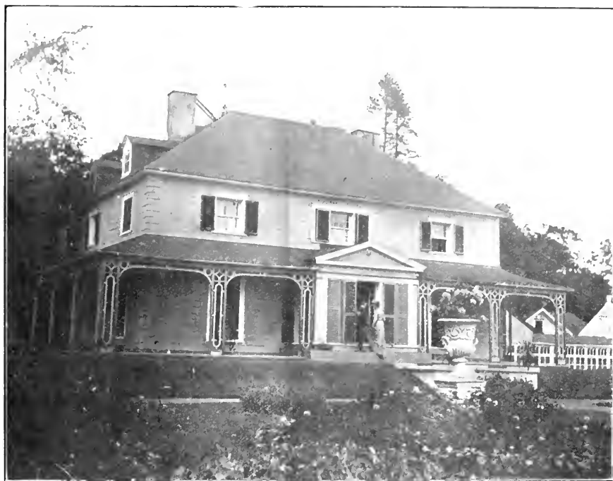
SPENCER GRANGE RESIDENCE OF SIR JAMES LEMOINE
